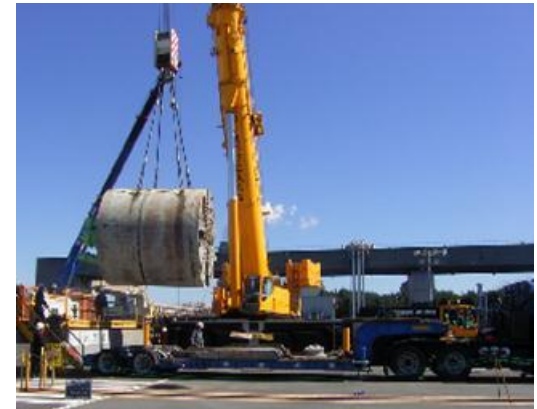
Taking out shield machine from tunnel
