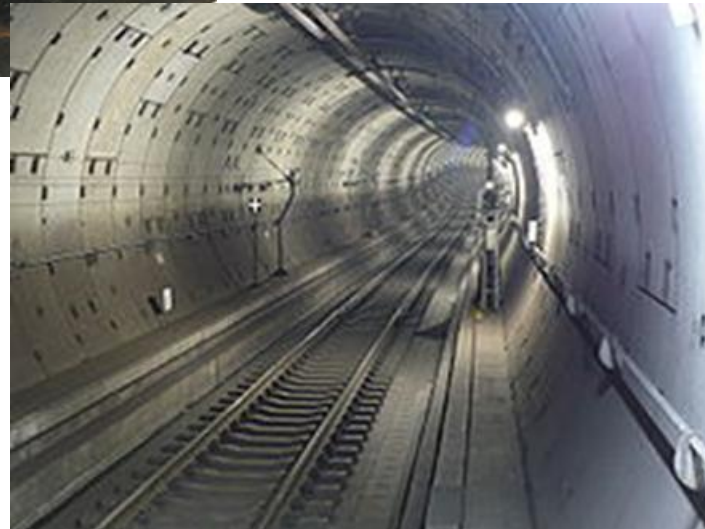
Underground construction of tunneling shield
